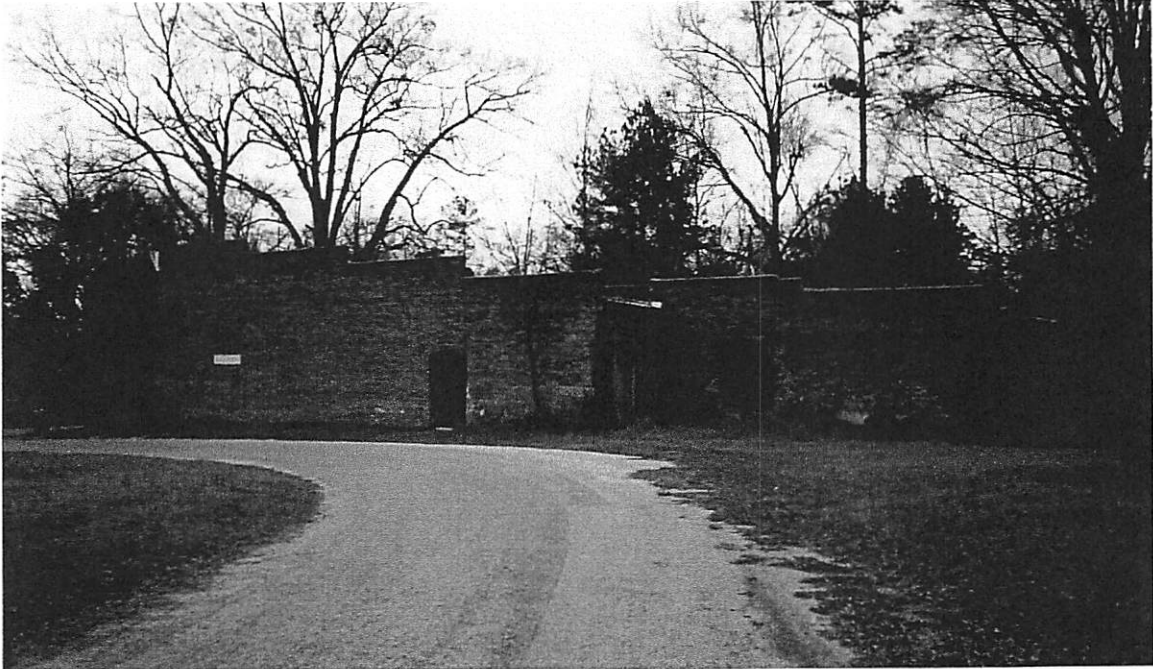
The side of the Durham Mercantile Company. The large door to the far right is the loading dock where farmers would load supplies into their wagons and where Mr. Durham would take in goods brought by train.
